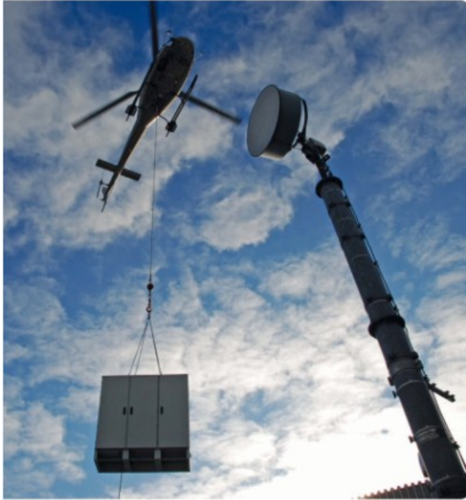
Airbus Defence and Space has used helicopters to get base station equipment to remote sites
